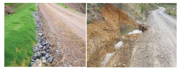
Figure 15 Example of energy dissipation rip rap (left) that will be employed in steep grade areas within the channel; and a sediment trap (right) that may be dug upstream of culverts. (Source: NZ Forest Road Engineering Manual).
