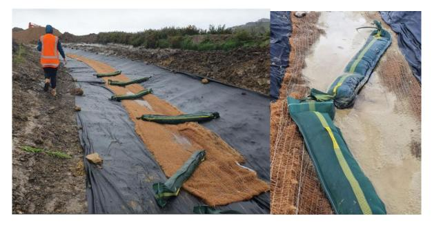
Figure 13 illustration of K-log channels and natural fibre matting successfully retaining fine sediment. (Source: EnviroCo)
