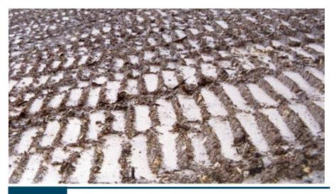
Surface roughening of a slope. Note that the hollows act as 'micro' sediment traps
