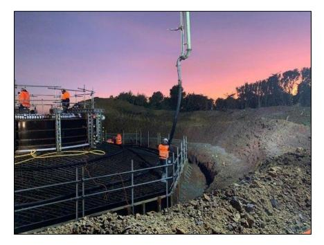
Figure 15 Example of a Tower Foundation Concrete Pour
